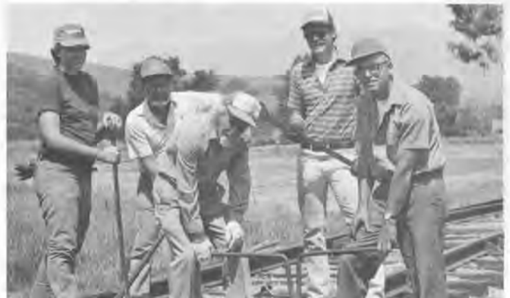
Gandy dancers pose during track-laying.
