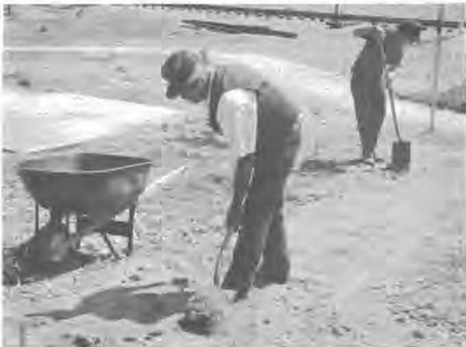
Al Jaramillo and Bill Parker work on path construction.
