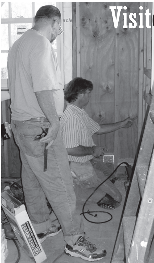
David Chapman and Daniel Moosbrugger prepare for the electrical installation.
