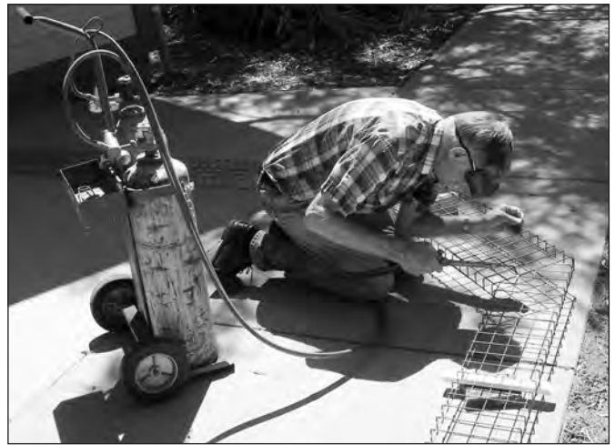
John Green welds together sections of the suspended railroad's supporting structure.
