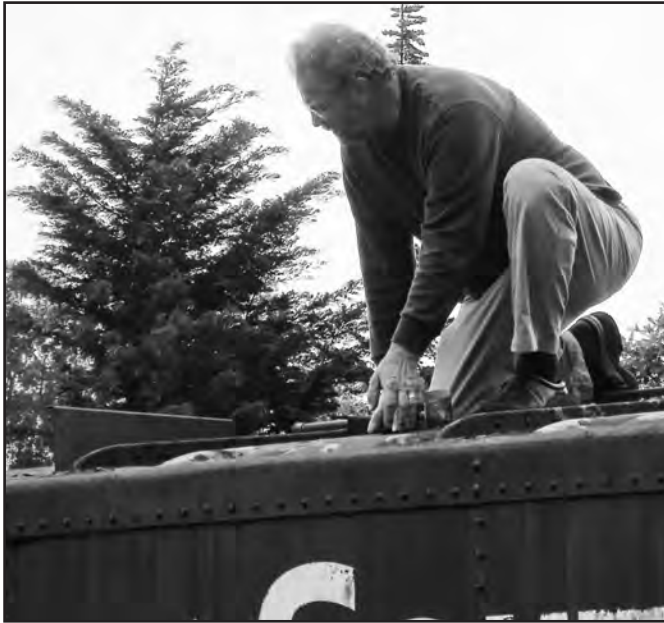
Conservator Brian Howard inspects the roof of No. 4023.
