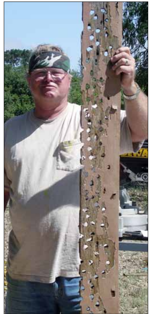
Builder Tom Brown shows woodpecker-damaged trim board from Goleta Depot.
